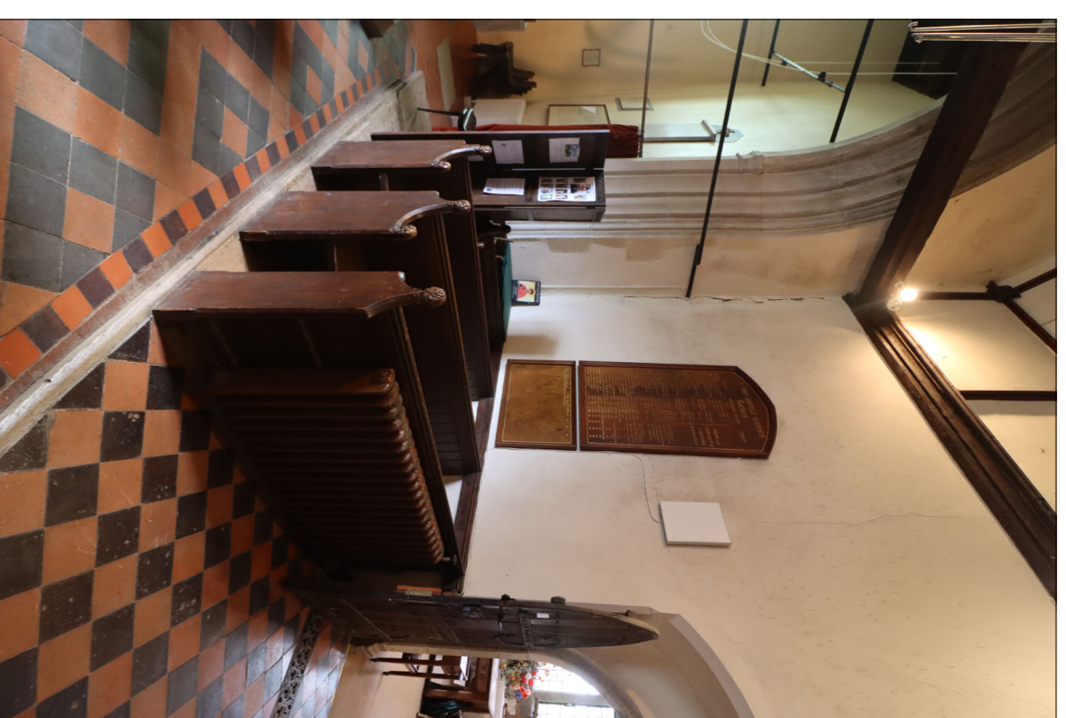
1 Location of existing pews and pew plinths that are to be removed, and wall-mounted elements such as the rector memorial boards and hearing loop box to be moved to accommodate new servery.
