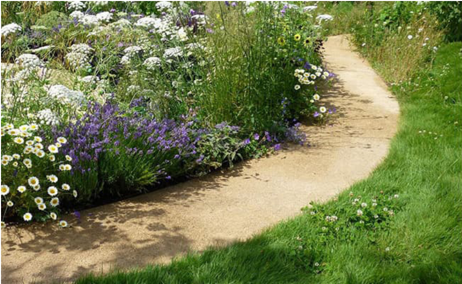
Proposed Self-binding Permeable Gravel Path to create compliant, but informal path into west door
