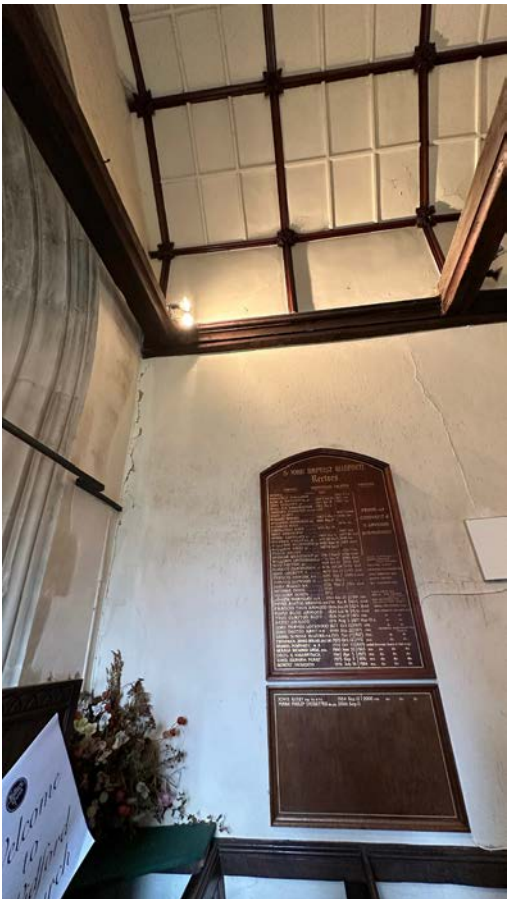
24. The ceiling of the wagon roof and the redundant beam next to the west tower arch
