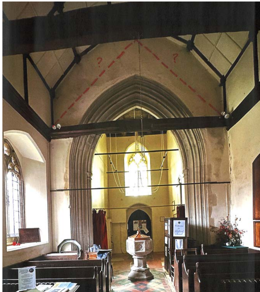
16. The possible 'lower' roof pitch at Widford before the raised heightened wagon roof was erected (see also the roof profile at local Hunsdon Church. All 7 facets of the wagon roof are equal in size at Widford).
