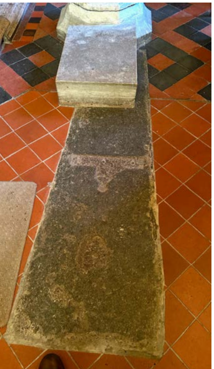
A west tower ledger stone obscured by a concrete step that has become a trio hazard
