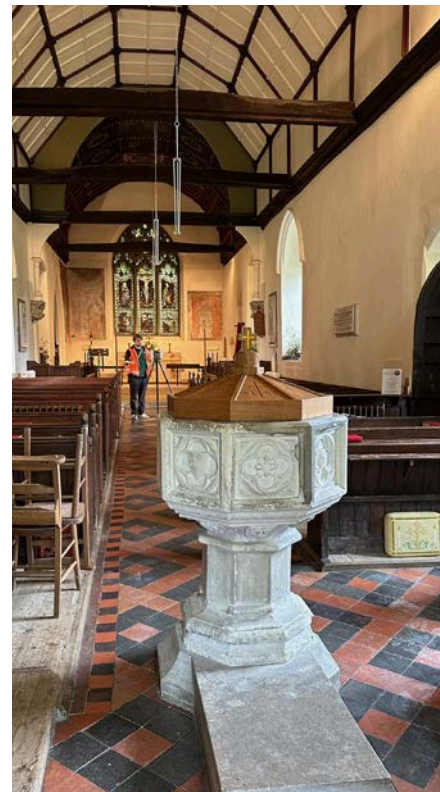
The font with added incongruous concrete base to be removed
